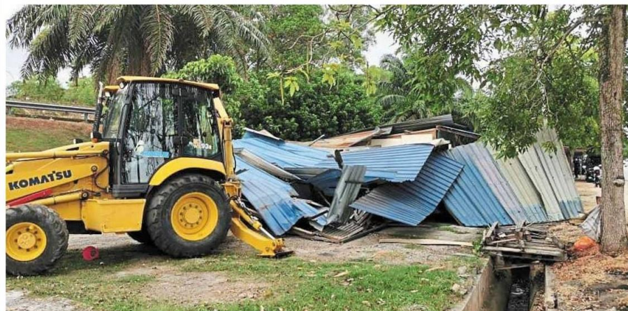
MBSJ's team demolishing one of the illegally built structures along the kerb of a main road in Kampung Bukit Lanchong, Subang Jaya.
