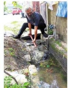
Tan showing the amount of mud in the drain along Lorong Batu Unjur 3A.
